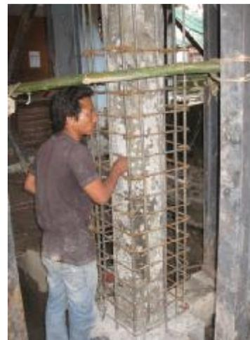
*Figure 4 – Reinforcement of column and anchoring bars*
