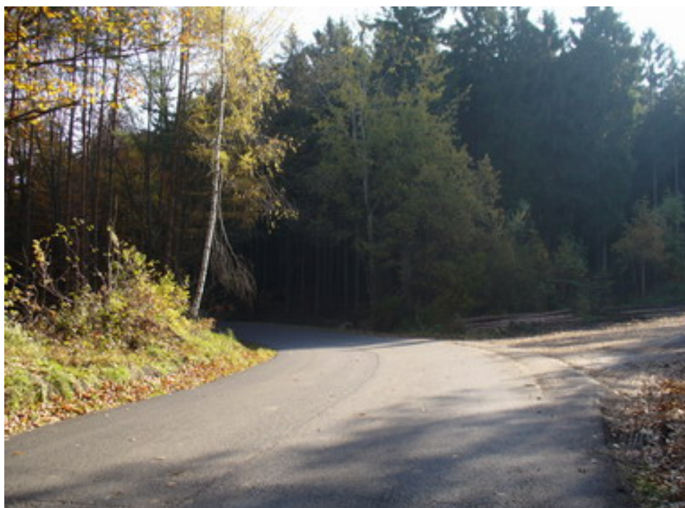
Figure 4 – Detail of the problematic place (intersection of road and forest path) (source: author)
