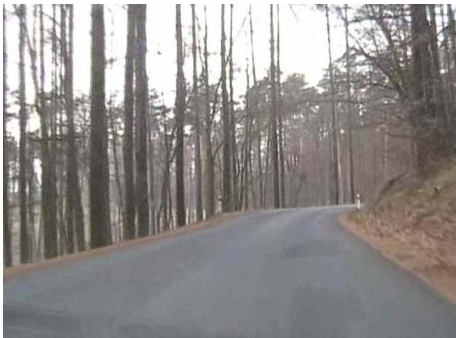
Figure 5 – Insufficient contrast of bend signs (source: author)
