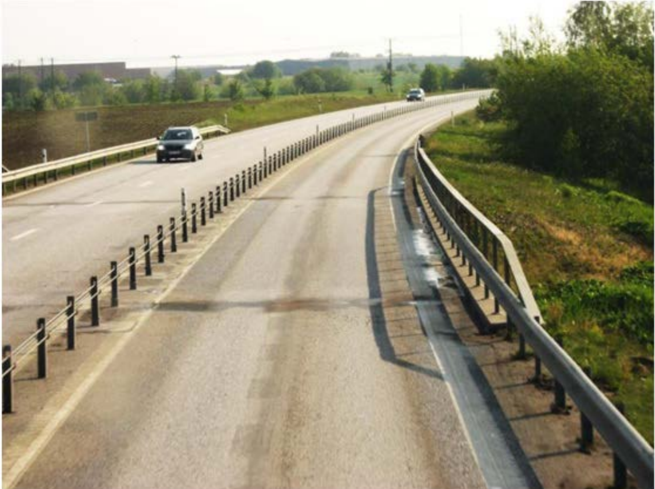
Figure 5 – Example of a 2+1 road with rope guardrail in the median [2]
