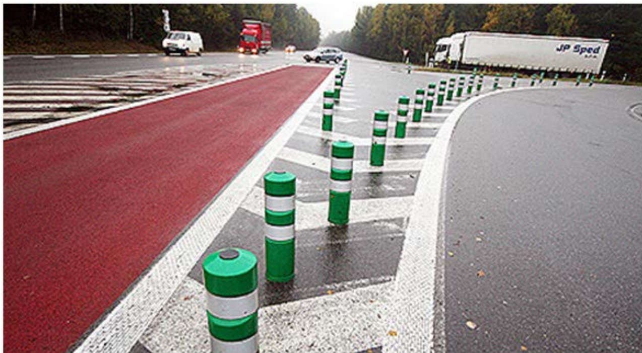
Figure 11 – Example of use of balisets (special green delineator post) used to emphasize the crossroads and which could potentially emphasize the changeover as well [5]
